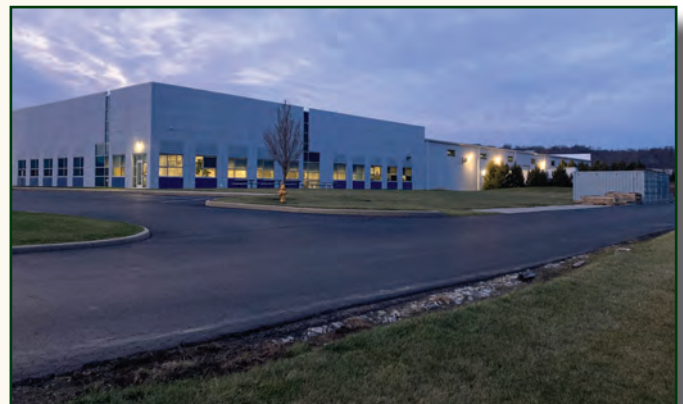
Photo above: Cincinnati Testing Systems in the City of Harrison, Hamilton County, Ohio
