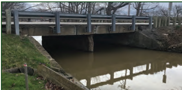
Photo shown above: Existing Westville Lake Road Bridge
