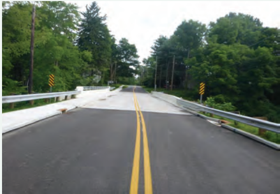
Photo above: Liberty Street Bridge road view
