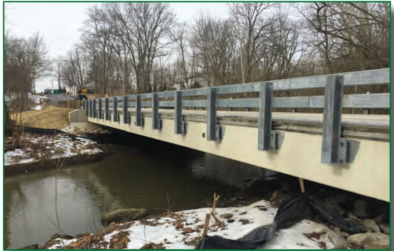
Photo above: MED-CR 78-0.91, Kennard Road Bridge in Medina County
