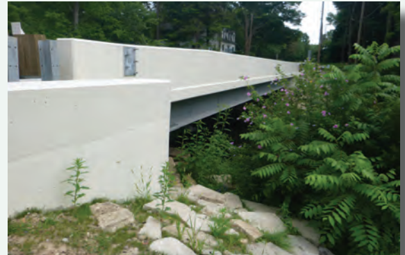
Photo above: Liberty Street Bridge side view
