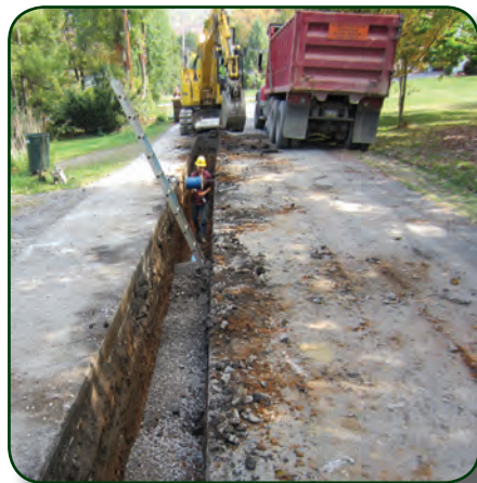
Photo above: Bellwood Borough Waterline Replacement Project
