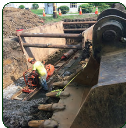
Photo below: Upper Tyrone Township Sewer Project
