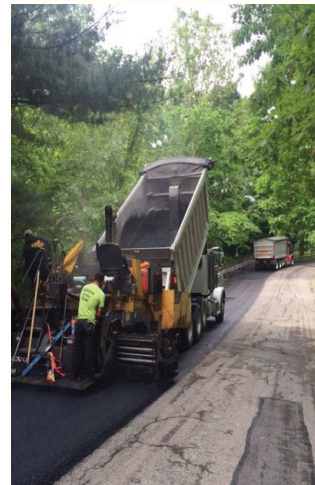
Photos above: 2017 Summer Paving Project in Murrysville, PA.
