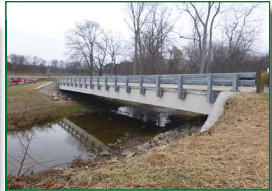
Photo above: Knox County - Thayer Road Bridge
