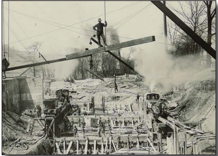
Photo above: Panoramic view showing the construction of concrete pump-pit, Ross Pumping Station, April, 1906
