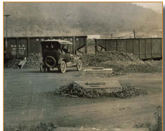
Photo above: Water Works Pumping Station showing the constructed manhole tops in February, 1927
