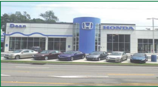
The Dean Honda project in 2014 located in Pleasant Hills, PA involved MKA providing surveying and civil site design.
