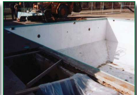
Photo above: 1980 - 1990 swimming pool inspection and restoration for Pittsburgh Municipal Pools
