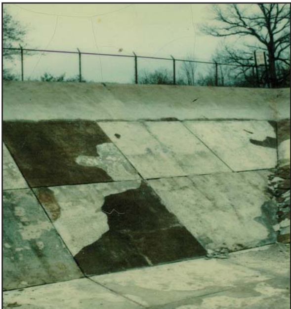
Photo above: In 1976 and 1977 Morris Knowles provided an inspection review and designed upgrades for the Zelenople, PA water reserves.
