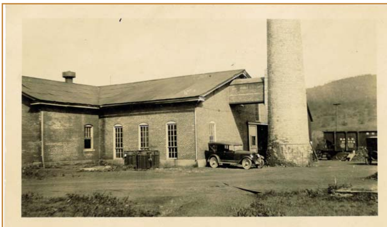
Photo above: Water Works Pumping Station in Franklin, PA. in October, 1926.
