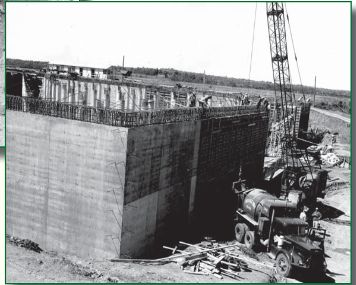
Photo below: The Construction of the Covered Reservoir for the Wilkinsburg - Penn Joint Water Authority.
