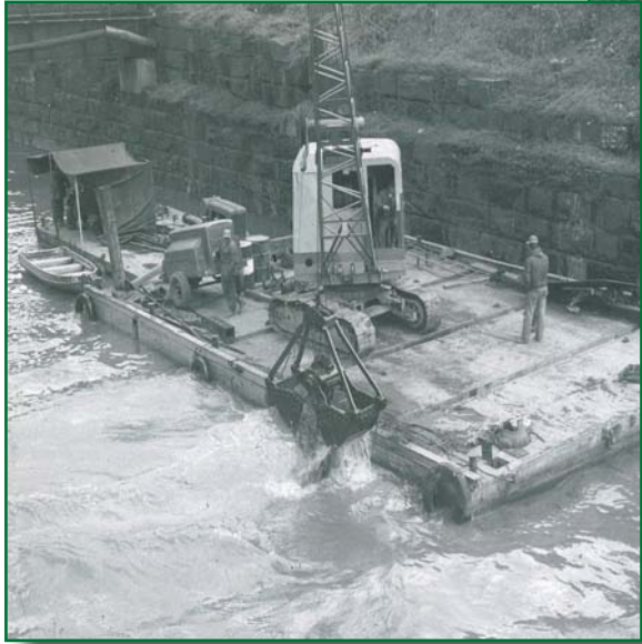
Photo above: Wilkinsburg - Penn Joint-Water Authority Excavation for a 16" line at Turtle Creek, PA in April, 1962
