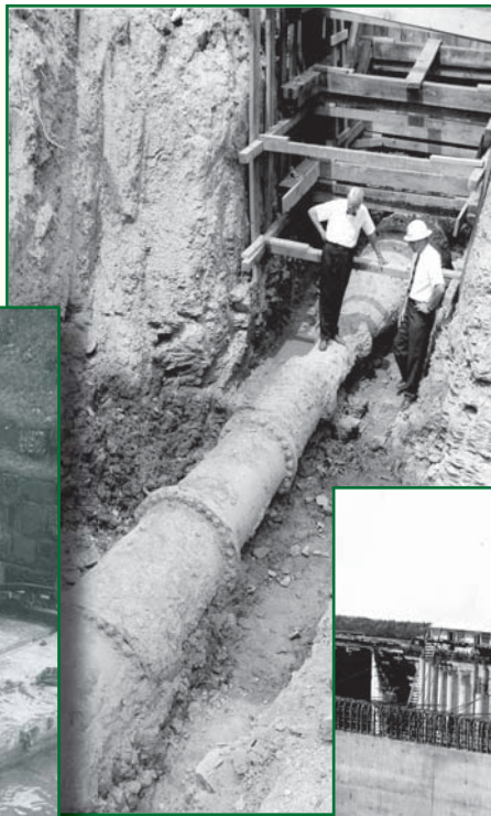
Photo left: The filter plant excavations for the 36" connection to a 42" line at the Wilkinsburg- Penn Joint Water Authority.
