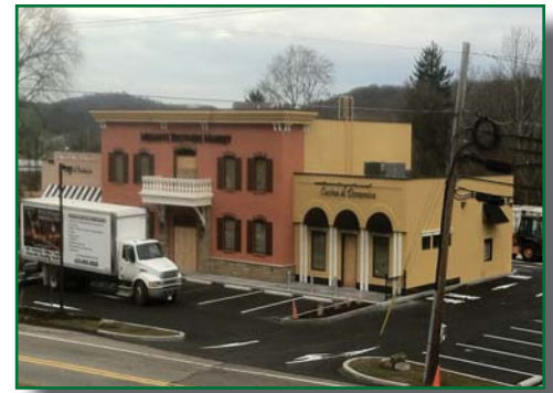
MKA was hired by Sweeney Shank Architects in 2012 to provide structural design services for the Mercante Brother's Market in Washington County, PA.
