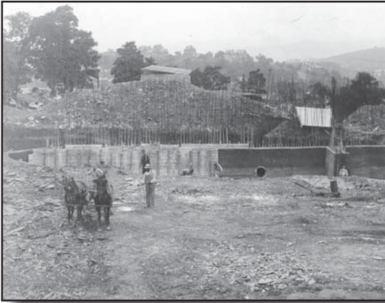
Photo above: Horses used in August 1909 to move equipment for the foundation of the Ross pumping station in Aspinwall, PA.
