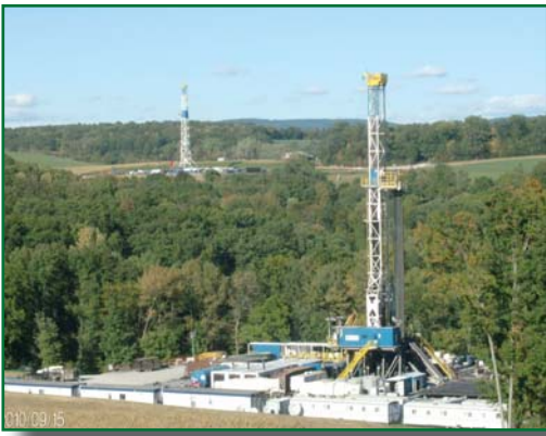
In the 2000s MKA began providing civil engineering and surveying services to oil and gas companies in the Marcellus Shale Play. Above photo: Marcellus Gas Wells.
