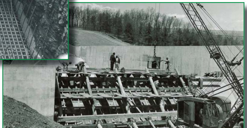
Photo above: Penn Forest Dam, Control Tower footing
