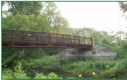
Photo left is the New Ligonier Valley Walking Trail Bridge. MKA served as Ligonier Township's Consulting Engineer on this bridge in 2012.
